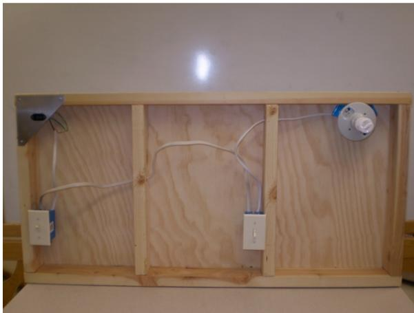
a. Three Way Switch Circuit
