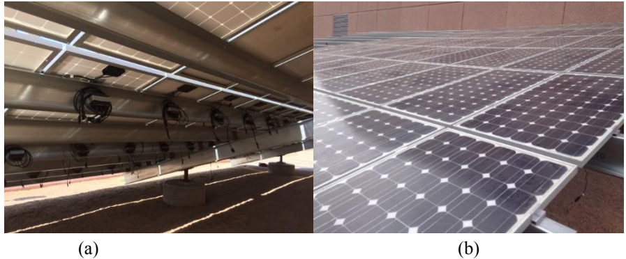
Fig.1: The Cyber physical (CPS) system allowing transmission of analytics and enabling the control of the system from remote sites. The figure shows (a) Solar array research facility with SMDs attached on each panel. (b) The SenSIP solar array facility. The educational value of this CPS facility is that students can learn about sensors and sensor fusion, the use of machine learning to optimize solar energy production.
