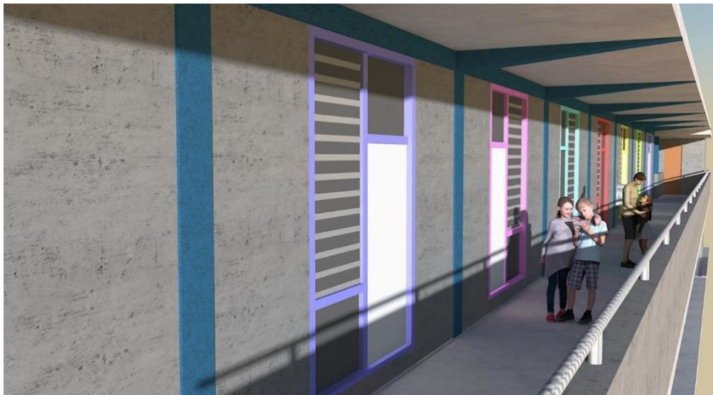
Figure 5- Exterior view with facades modifications. From [8].
